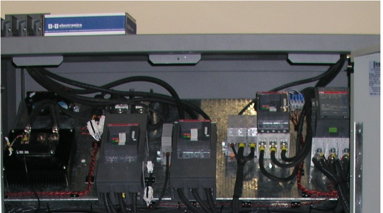
Figure 7b When Inverter Drive Unit is on Center Shelf (No input Terminal Block)
